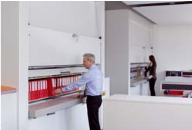
A fire-retardant door at the access point gives the files optimum fire protection
