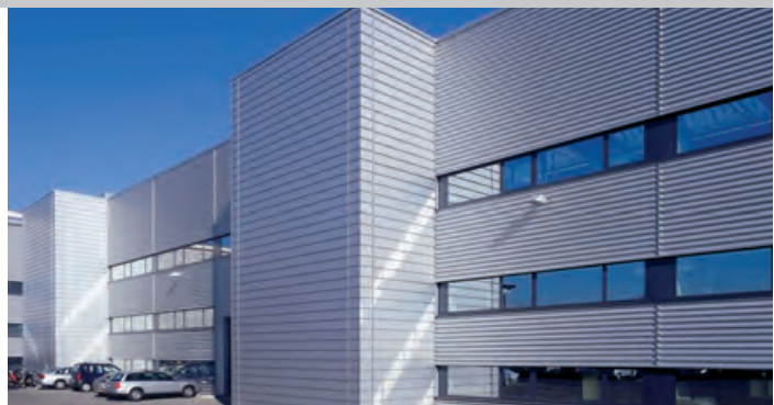
Two groups of Lean-Lifts® spanning multiple floors were attached to this building from the outside – no production space was sacrificed
