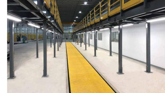
The integration of a mezzanine is an important component in the daily function of these facilities. To complete routine maintenance, trains must be accessible from both above and below. How can this be done safely?
