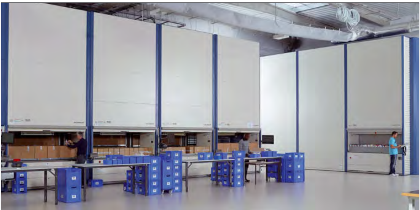
Storage of valuable electronic components for the aerospace industry at Air Cost Control in France
