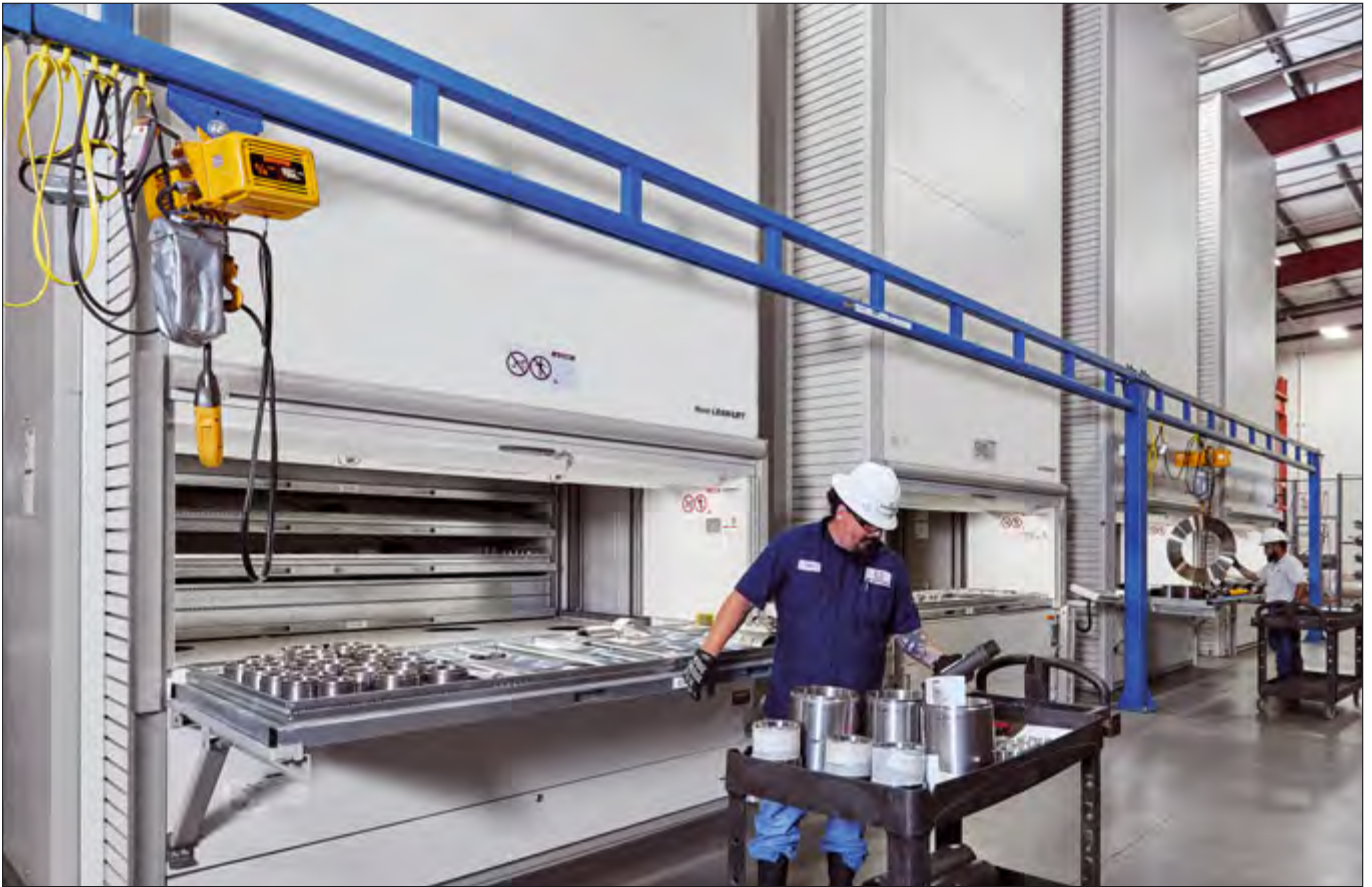
Storage of heavy components for the oil and gas industries at the TAM International production facility in Texas, USA
