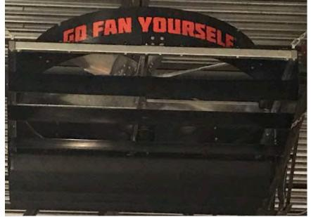
**TAZ FAN** is an industrial, two-directional fan that is ideal for spaces in need of an energy efficient targeted air movement solution. TAZ can replace four large single-speed, panel-aisle fans, or up to eight 36<sup>°</sup> basket fans while using only half the power. Adjustable louvers direct air for targeted cooling. Corrosion-resistant fiberglass housing and maintenance-free motor ensure a long life and covers over 5,000 square feet on high speed.
