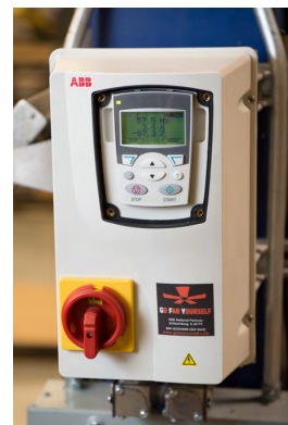
Fan Control ABB VFD With LOTO Disconnect (Found inside Motor Hub Assembly Box)
