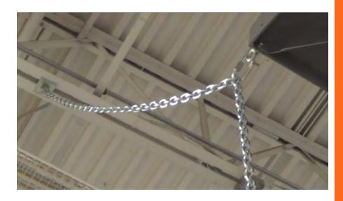
• Slowly lower the lift so the fan weight is gradually taken by the chain. The fan may swing as weight is transferred. Support the fan manually to reduce the potential swing to prevent possible damage to the fan.
