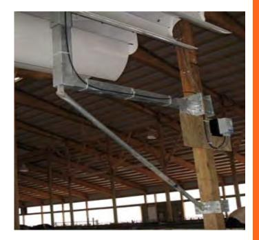
NOTE: For wall or column mounts the bracket will be required to be approximately 40" long. This bracket must be designed to support the 375lb fan. It must also be supported by a brace similar to shown in the pictures above and below. The bracket must also hold the 1250 ft lbs of twisting force created by TAZ at full speed.
