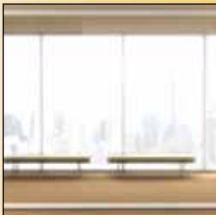
Unitized butt-glazing between panels makes unsightly vertical posts unnecessary.
